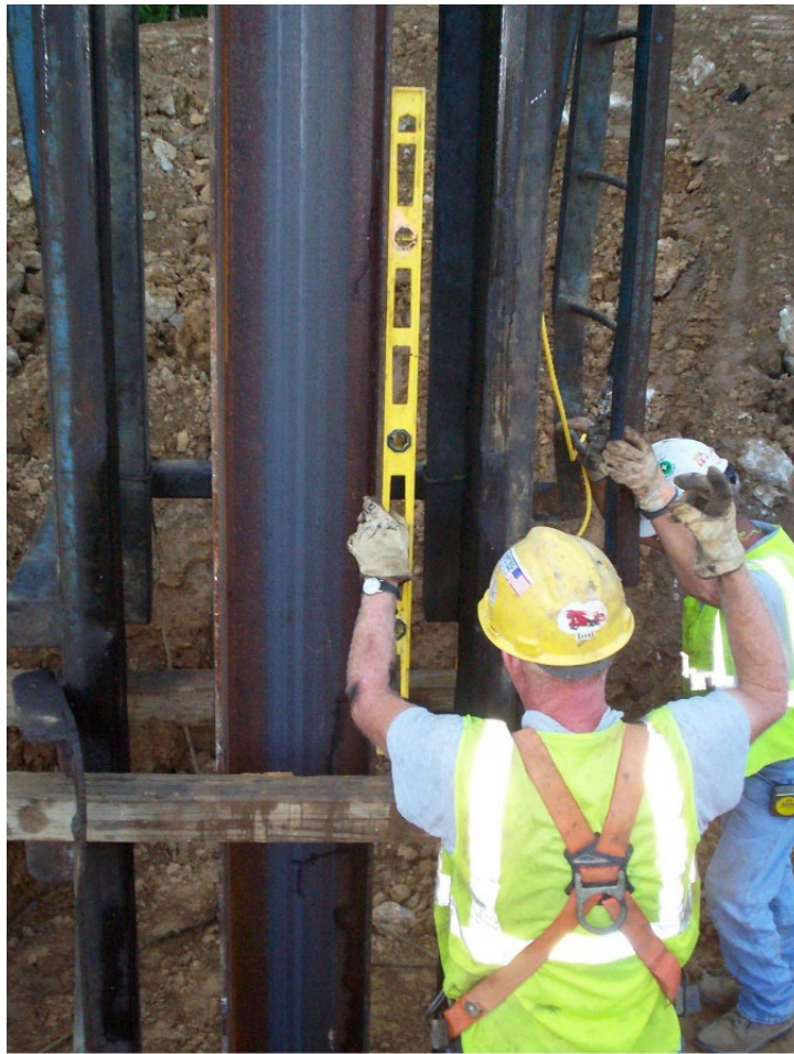
Figure 11 Contractor Checking Pile Alignment
