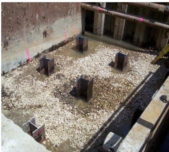
Figure 14. Piles cut-off at plan elevation
