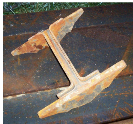
Figure 10 Top (Connection Side) of H-Pile Shoe Tip
